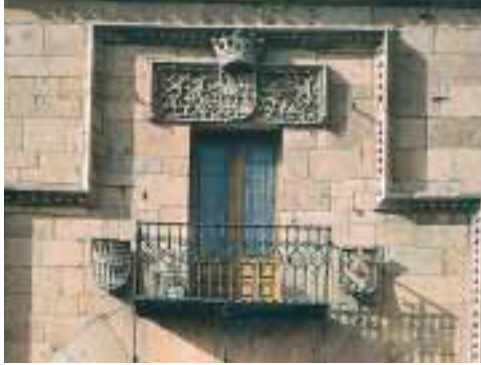
■ María la Brava's House. Detail of the façade.
